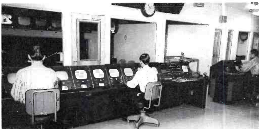
FIG. 14. TV Master Control. At left, Paul Wilson and George Alsobrook are at the video controls. At right, Mac Hix is at master audio console. Sub-control A is in front of video console. Master panel for TS-40 Switching System is at right end of video console.
